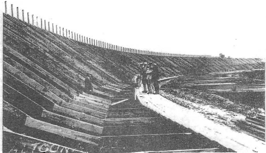
Constructing the track surface circa 1922 with its 40 degree banking. (Picture courtesy Jean Neely).
